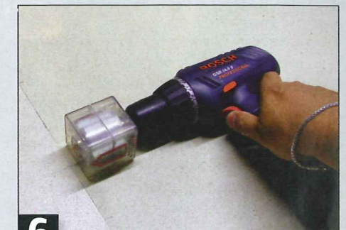
6 To complete the joint, set the drill to the correct orientation. The magnetic device winds the threads in
